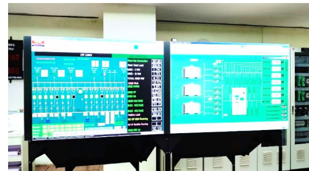
Installation of new BARCO make LVS
